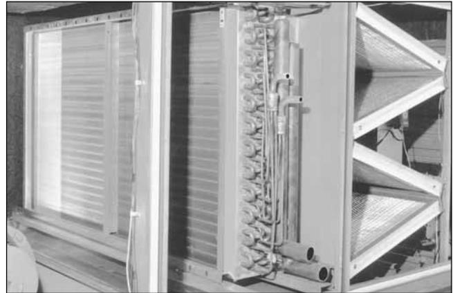
Please refer to tables 5 and 6 for Cooling Coil Performance Data. If a cooling coil is to be installed upstream of a duct furnace, a 409 stainless steel heat exchanger is recommended.
