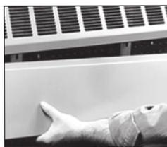
Draw one level chalk line on the installation wall and you're off to the races. Standard bracket is supplied with one or two adjustable element supports that allows a 1-1/8" vertical movement.
